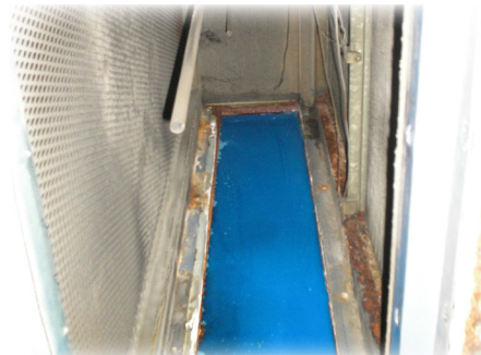
Completed polymer resurfacing
