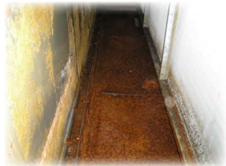
Cleaning of rust and debris
