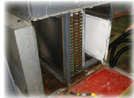
AHU unit prior to restoration
